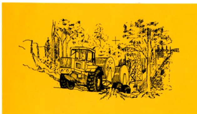
Equipped with dual cable laying rolls.
