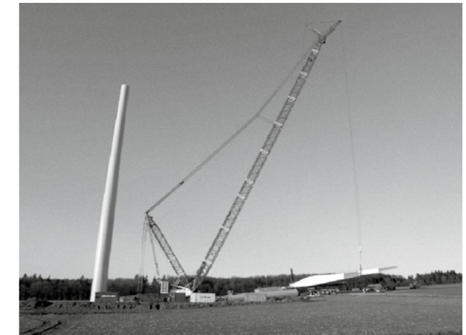
LARGE CRAWLER CRANE (Repower MM82 on 95 m tower)
