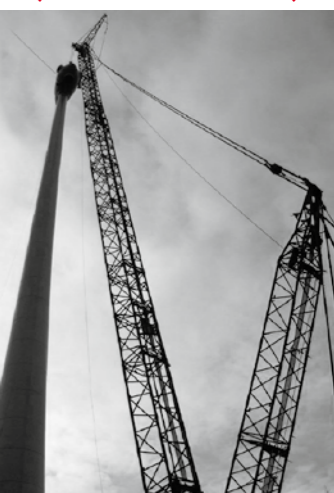
LARGE LATTICE MOBILE CRANE (Enercon E82 on 98 m tower)
