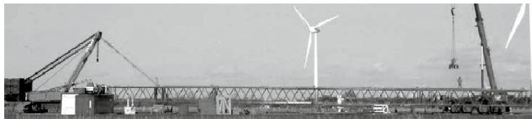
MEDIUM SIZED CRAWLER CRANE (GE70 on 98 m tower)
