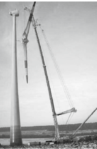
LARGE MOBILE CRANE (Enercon E70 on 98 m tower)
