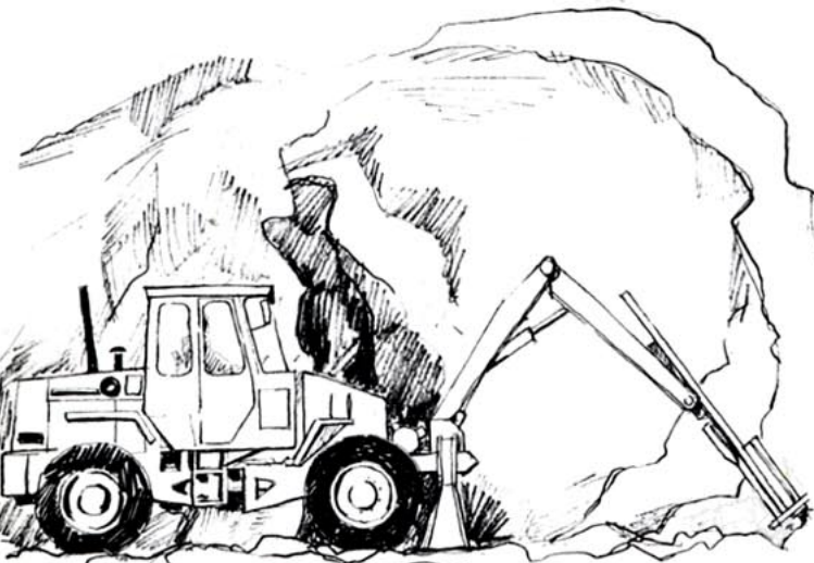
SPLITTING BOULDERS with water
