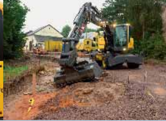
• All-around excavator/tool-carrier performance.
