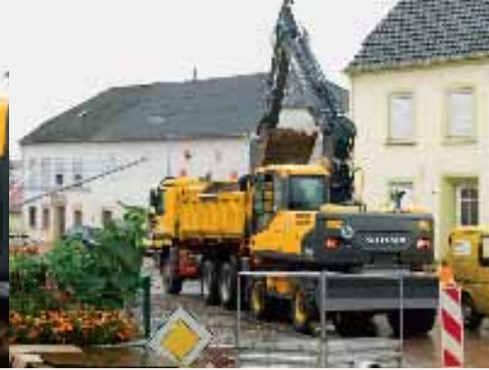
• Reach and power for digging and loading.
